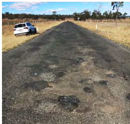
Jack Smith Gully Road – before
