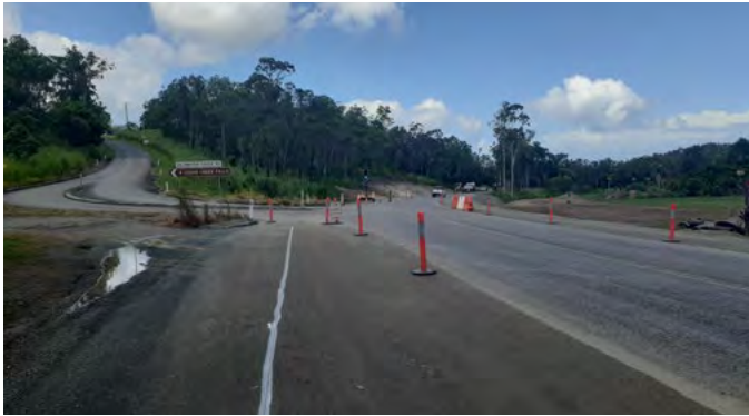
Conway Road – before
