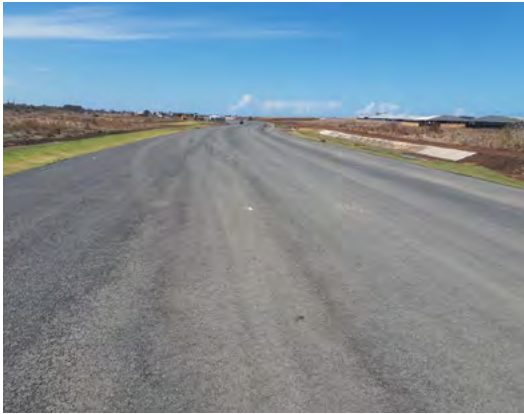
Hughes Road Extension (Watsons Road to Wearing Road) - works
