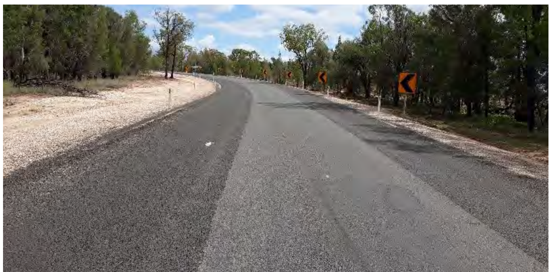
Auburn Road – after
