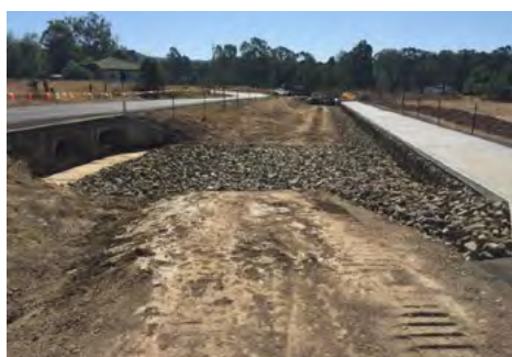
Murphy's Creek Road – construction
