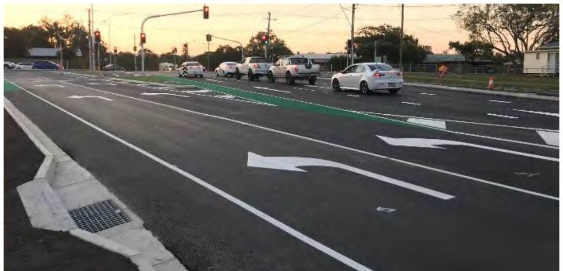
Oakey Flat Road/Walkers Road Intersection – after
