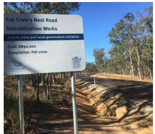
Crows Nest Road – project signage
