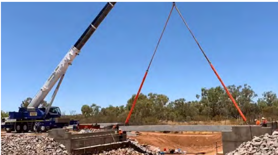
Carl Katter Bridge – construction
