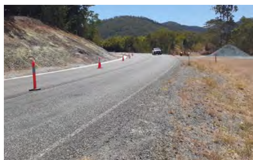
Conway Road – before
