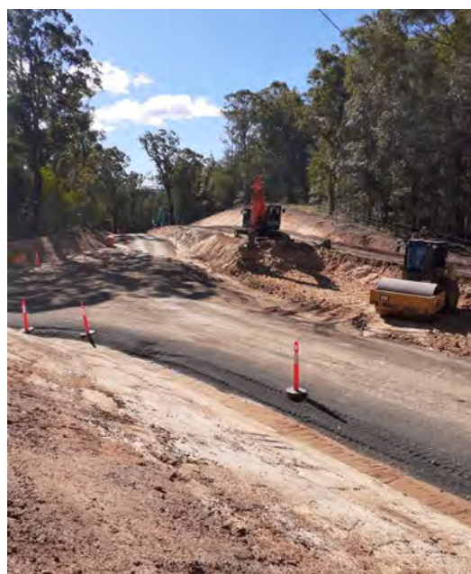
Beechmont Road – construction
