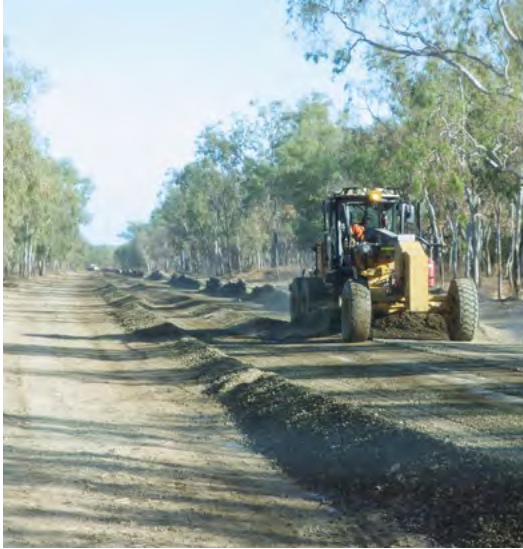
Topsy Creek Road – construction
