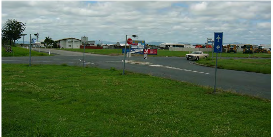
Milton Street and Boundary Road East Intersection – before
