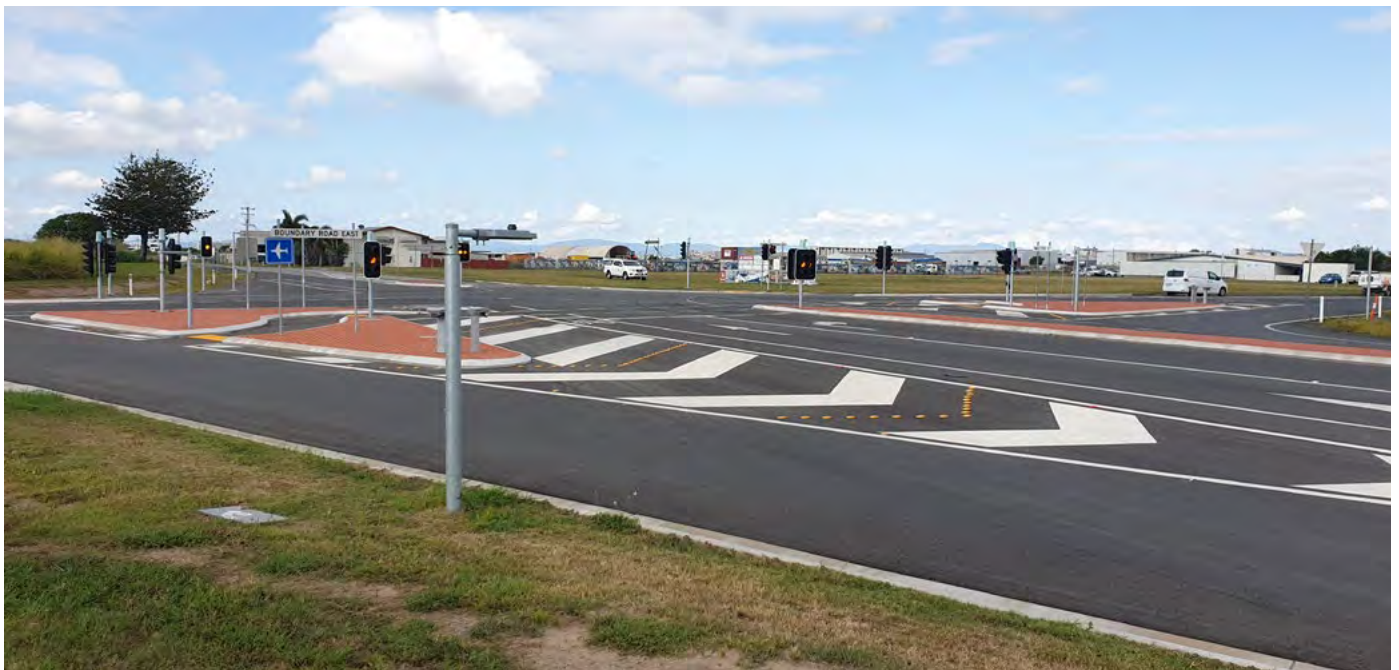
Milton Street and Boundary Road East Intersection – after
