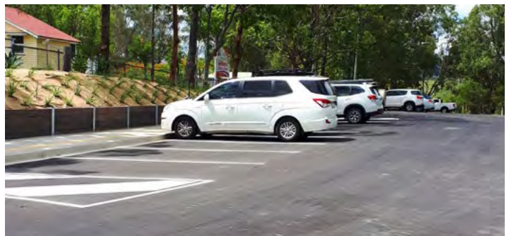
Glenwood State School Carpark – after
