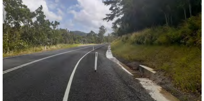
Conway Road – after
