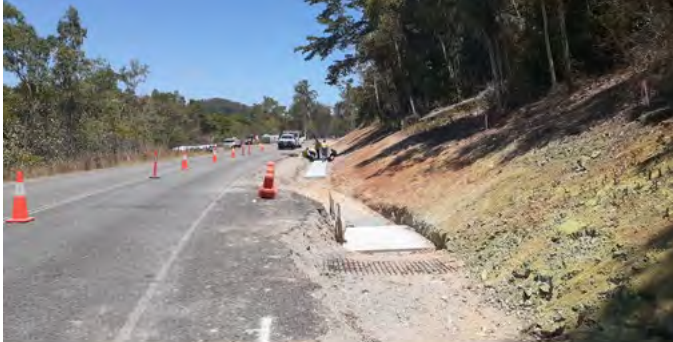
Conway Road – before
