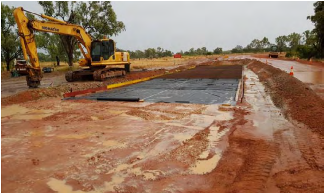
Strathmore Road – construction
