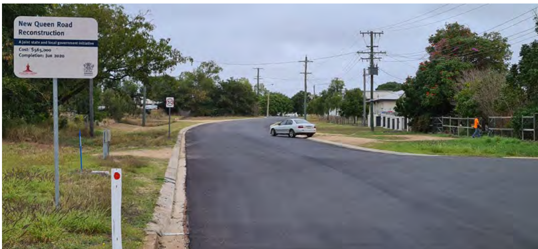
New Queen Road, Enterprise Road – after
