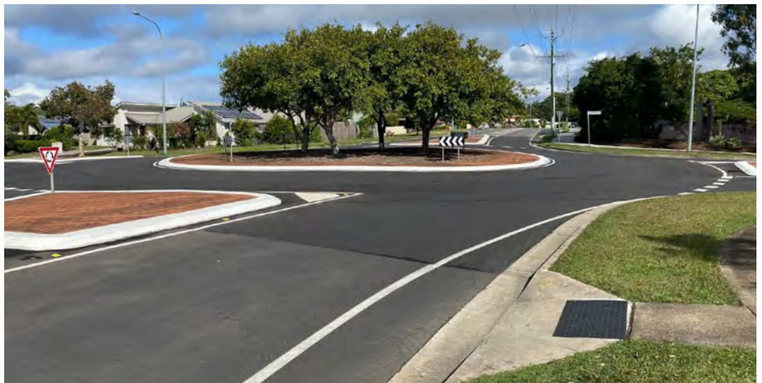
Bunker Road – after
