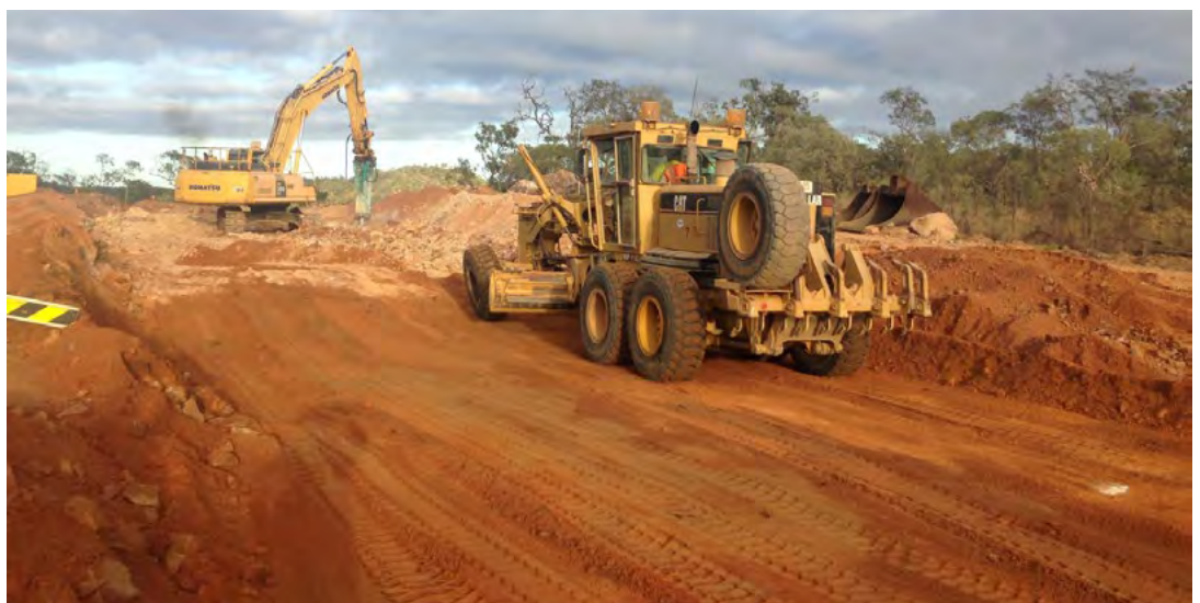
Ootann Road – construction
