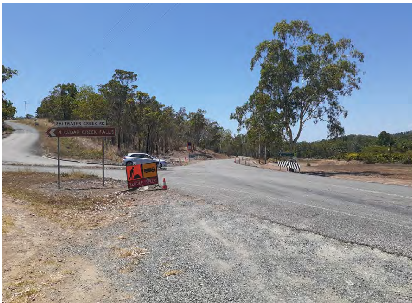
Conway Road – commencement of works
