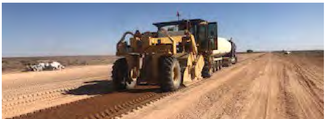
Eyre Developmental Road (Sunshine Flats) – before
