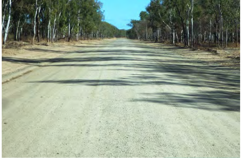
Topsy Creek Road – after
