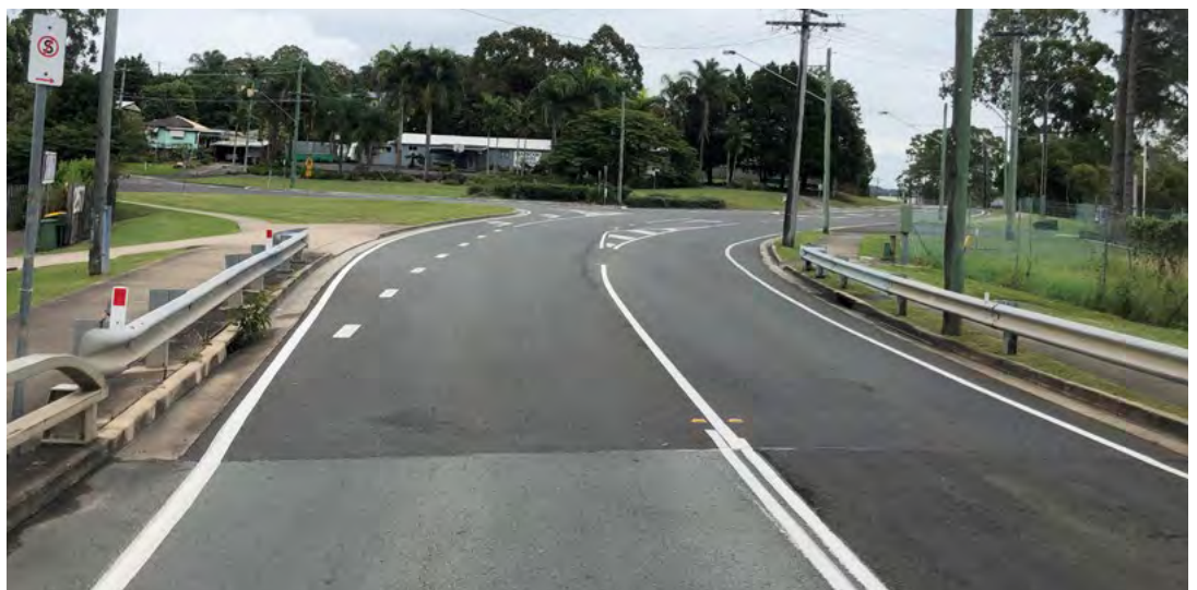
Main Road, Kuluin – after
