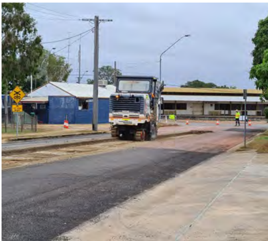
New Queen Road, Enterprise Road – construction
