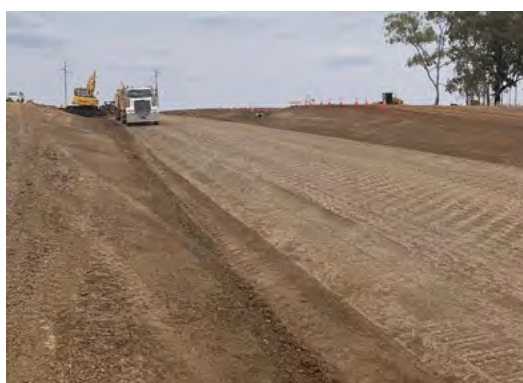
Jondaryan–Mt Tyson Road – construction
