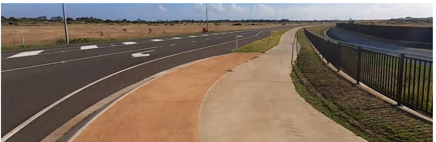
Hughes Road Extension (Watsons Road to Wearing Road) - footpath
