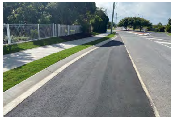
Bunker Road – after
