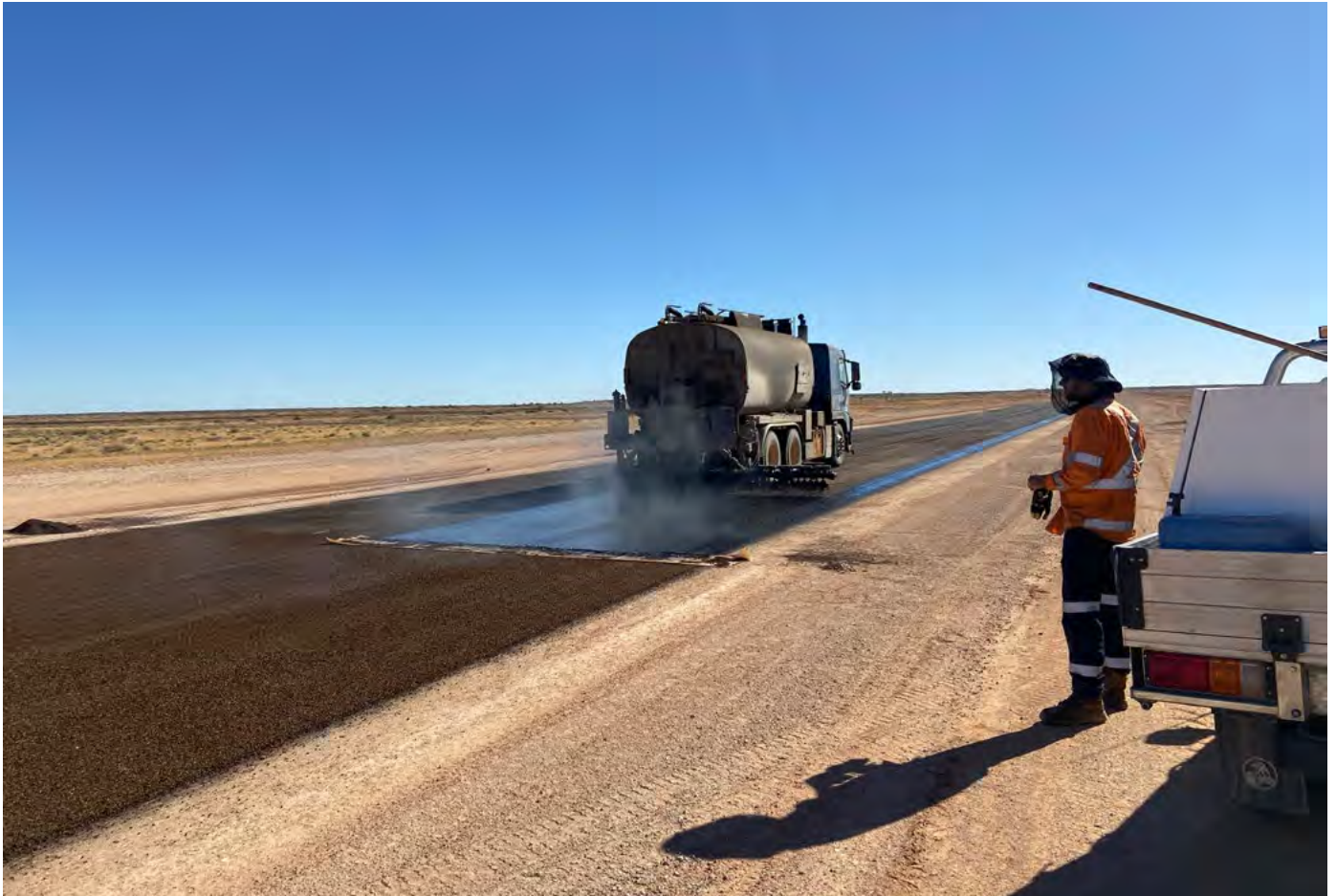
Eyre Developmental Road (Sunshine Flats) – construction
