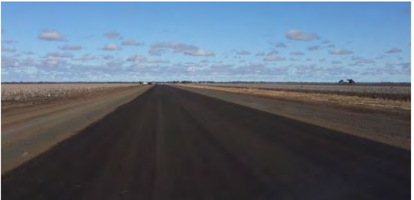
Jondaryan–Mt Tyson Road – after
