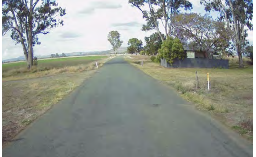
Van Itallies Road – before
