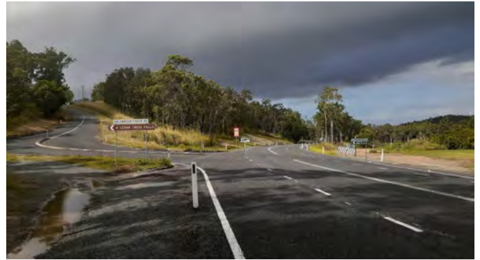
Conway Road – after
