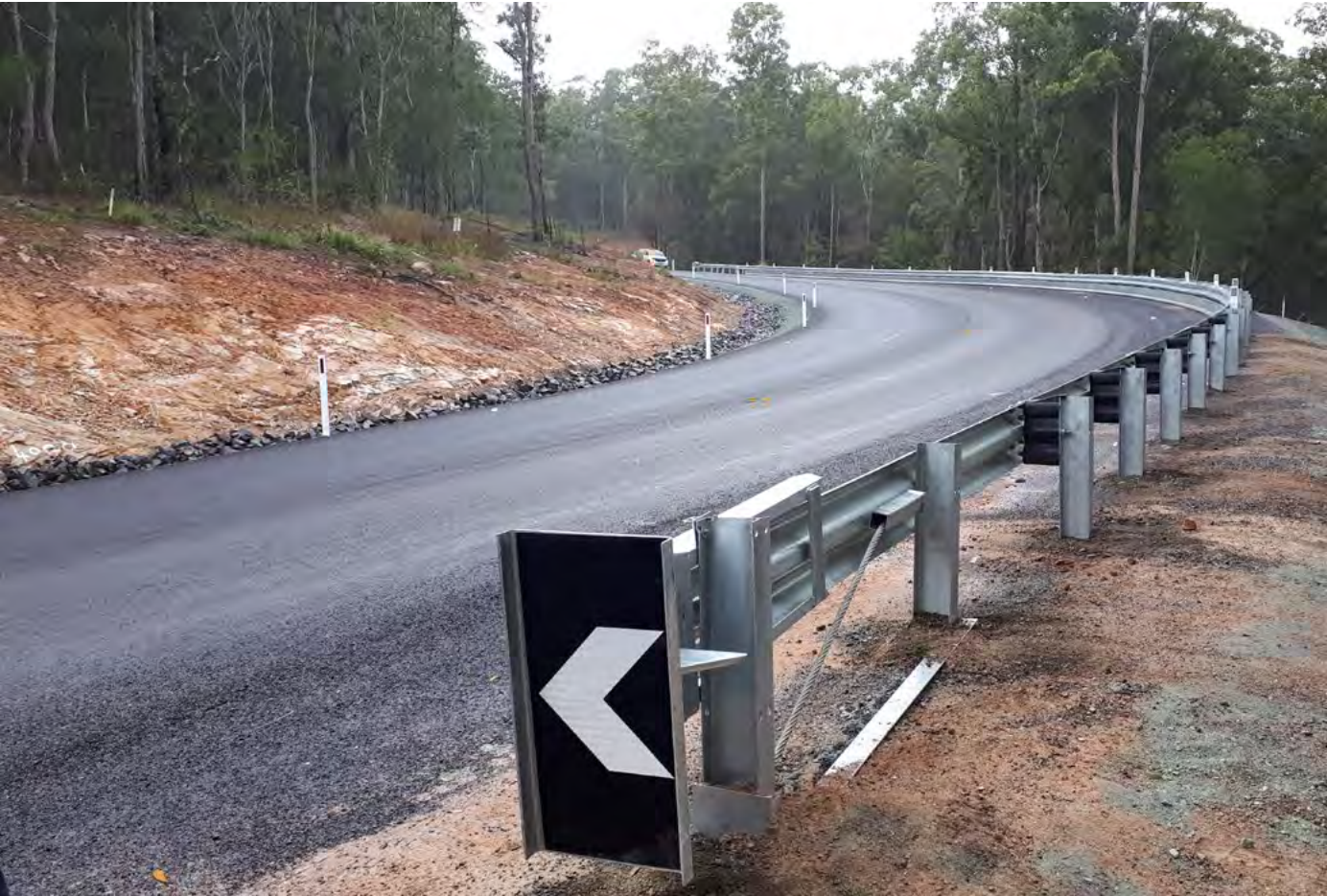
Beechmont Road – after
