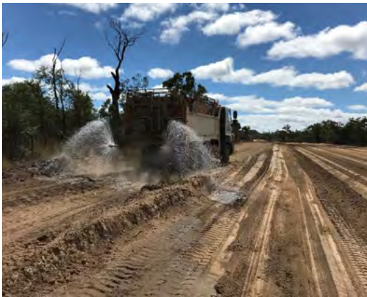
Ootann Road – construction
