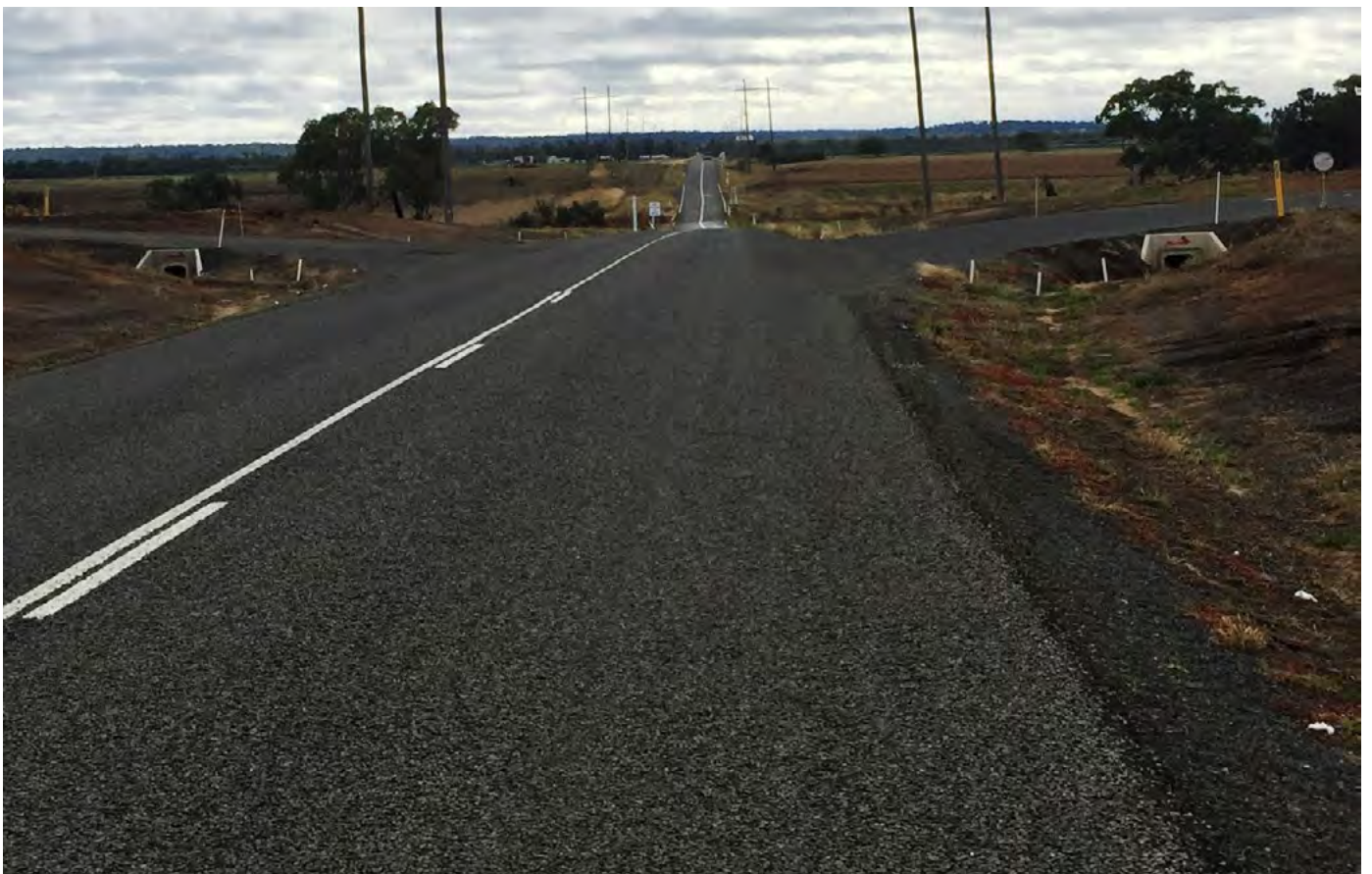
Jondaryan–Mt Tyson Road – after
