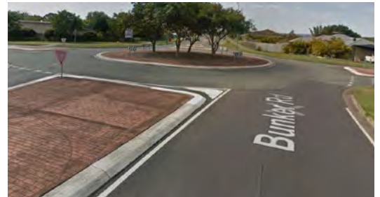
Bunker Road – before
