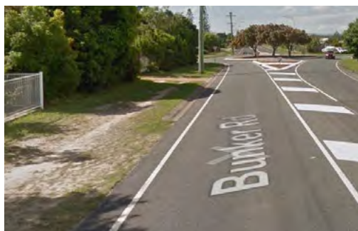
Bunker Road – before
