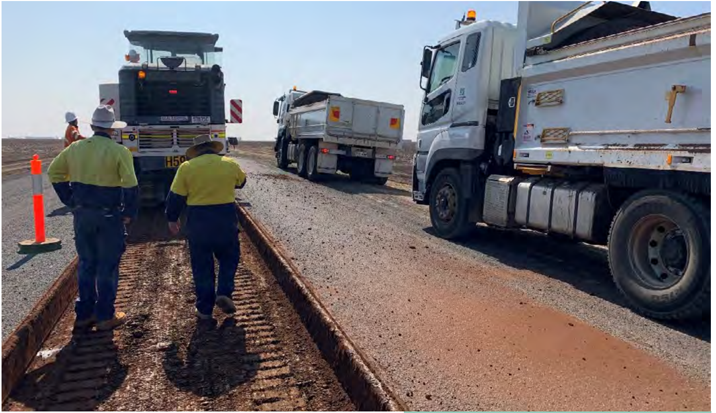
Jondaryan–Mt Tyson Road – construction
