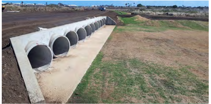
Hughes Road Extension (Watsons Road to Wearing Road) - works
