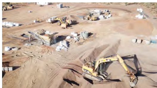
Woologarang Road – construction
