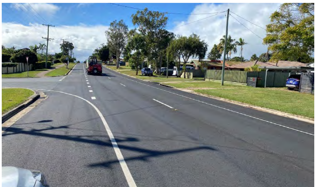
Benfer Road – after
