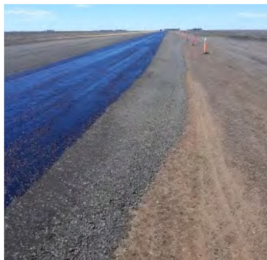
Jondaryan–Mt Tyson Road – construction
