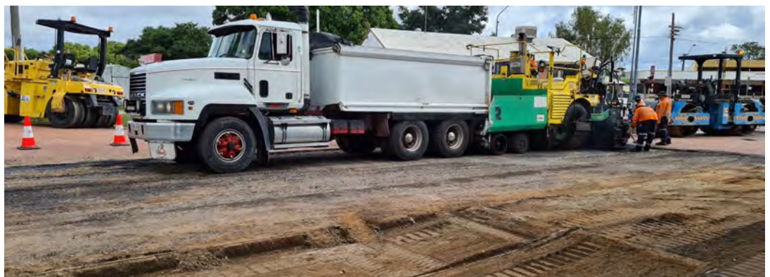
New Queen Road, Enterprise Road – construction
