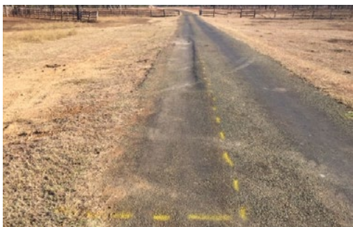
Blackboy Road – before
