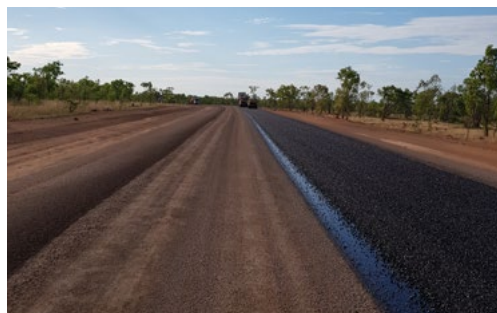
Strathmore Road – construction
