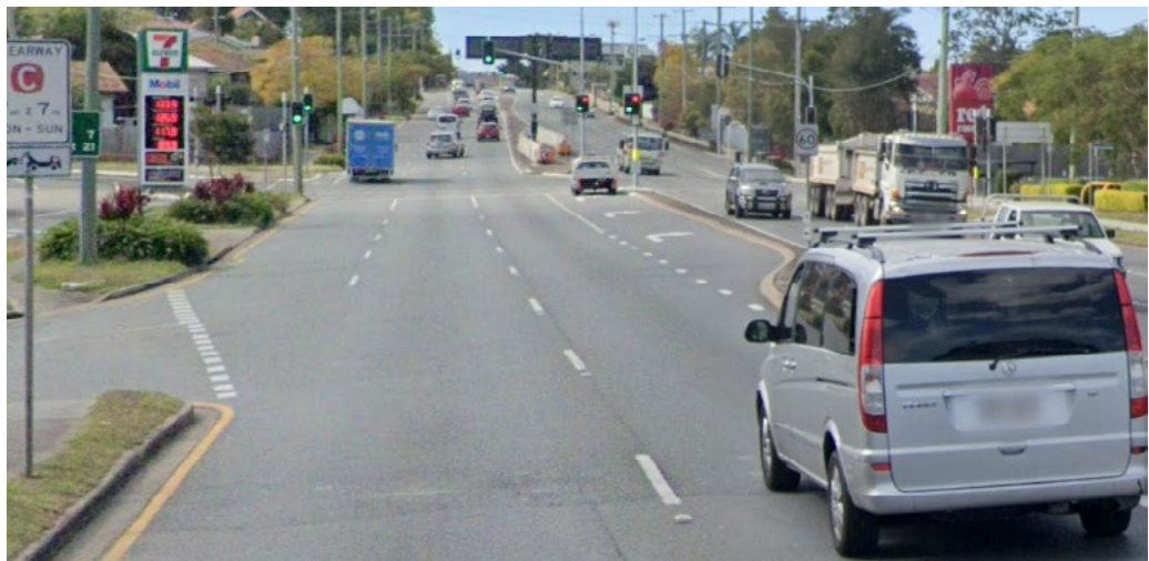
Ipswich Road – before
