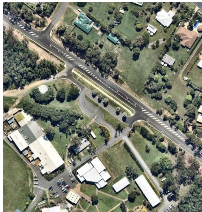
Adelaide Park Road – after
