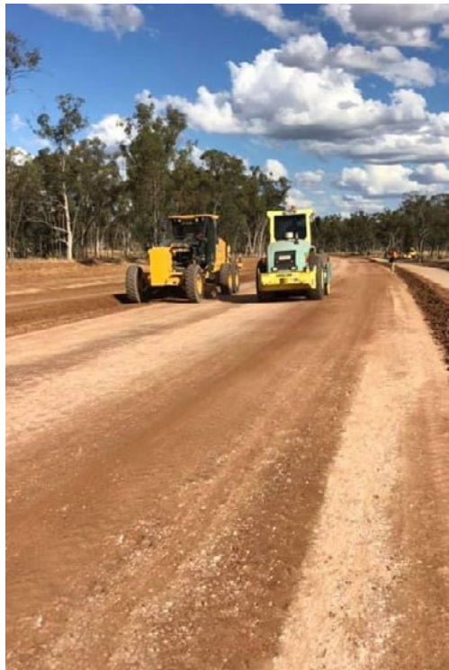
Alpha-Tambo Road – construction
