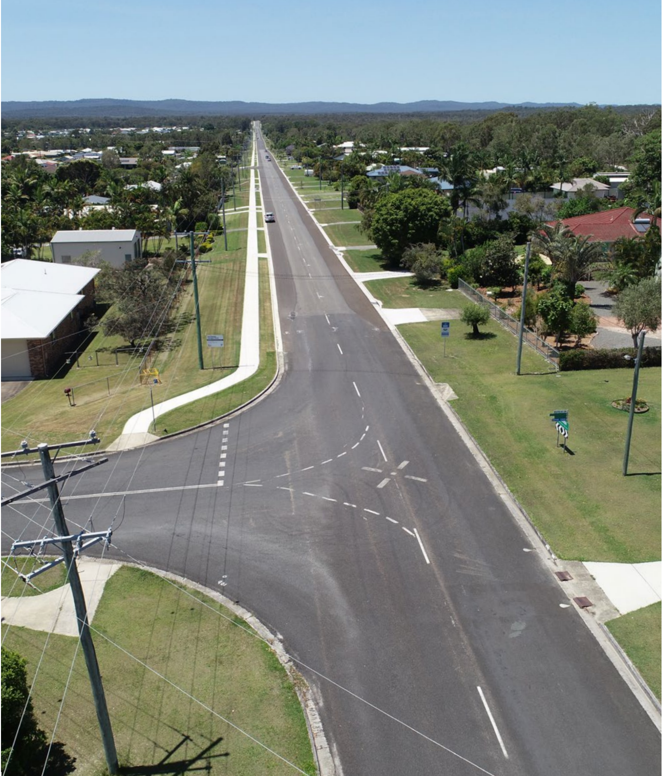
Investigator Avenue – after
