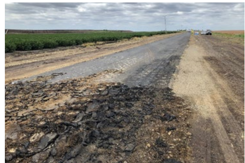
Bongeen Road – construction
