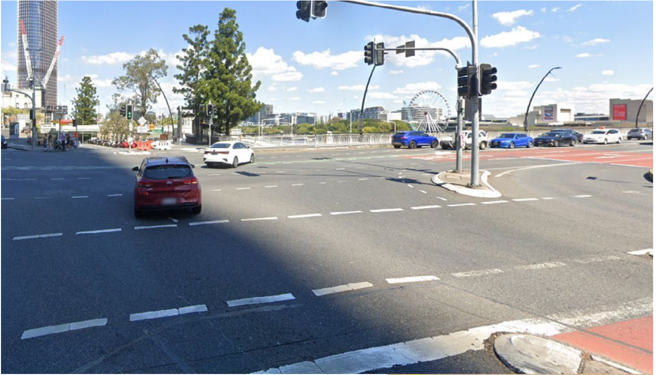
CityLink Cycleway – Stage 2, William Street to Gray Street – before
