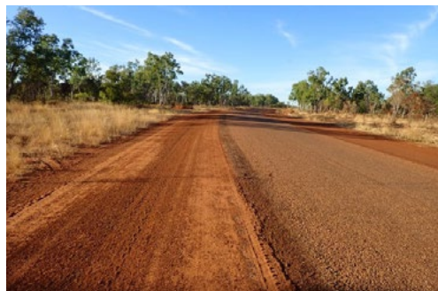
Woologarang East Road – before
