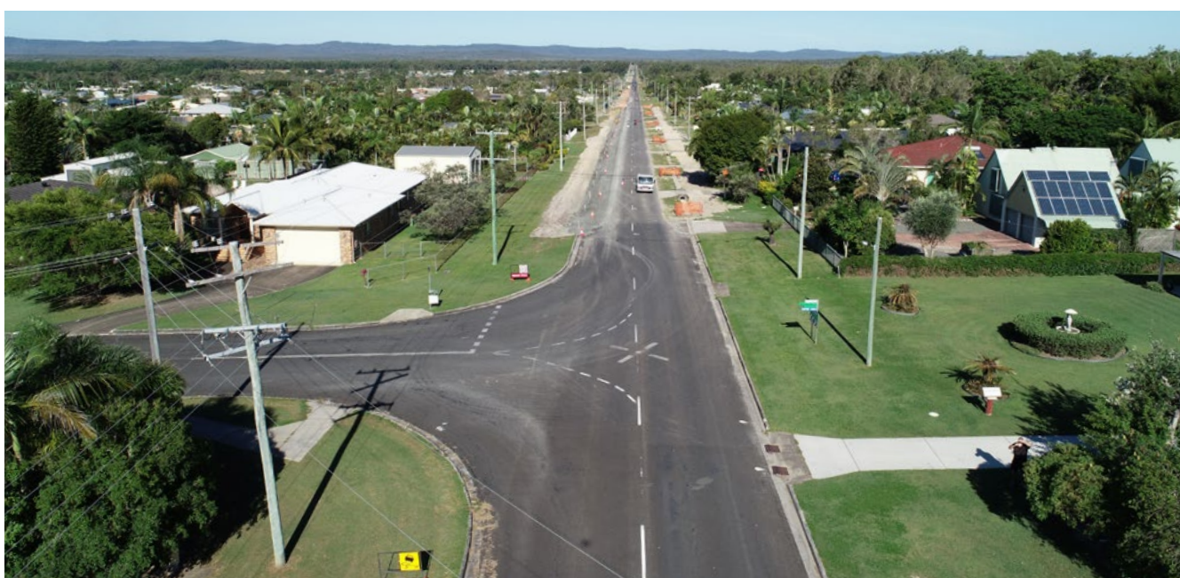
Investigator Avenue – before
