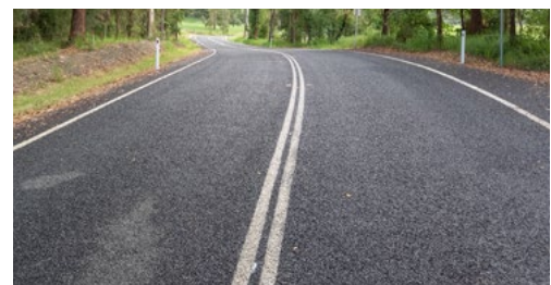
Kiamba Road – after
