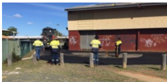
Kangaroo Stadium access – during
