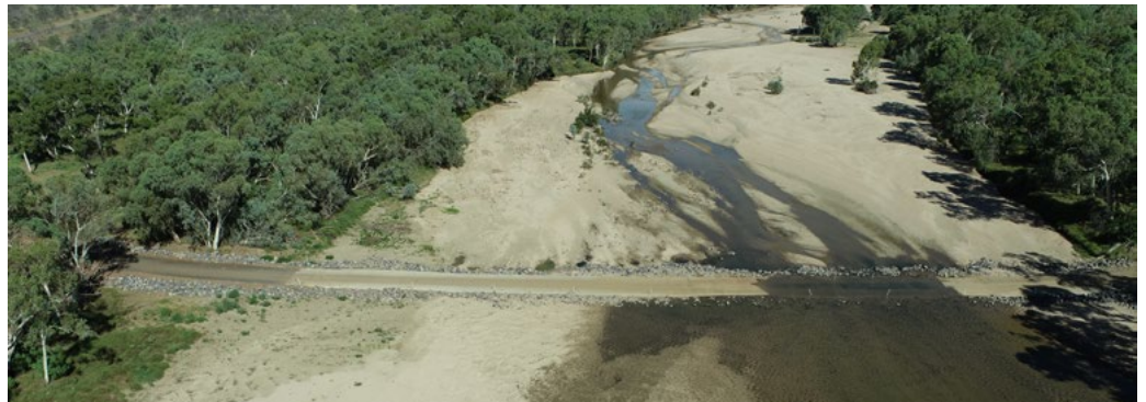
Glentor Road, Flinders River Crossing – completed
