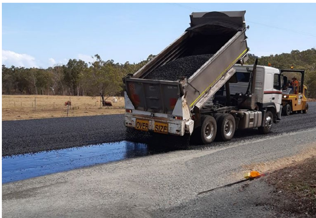
Ball Bay Road – during construction
