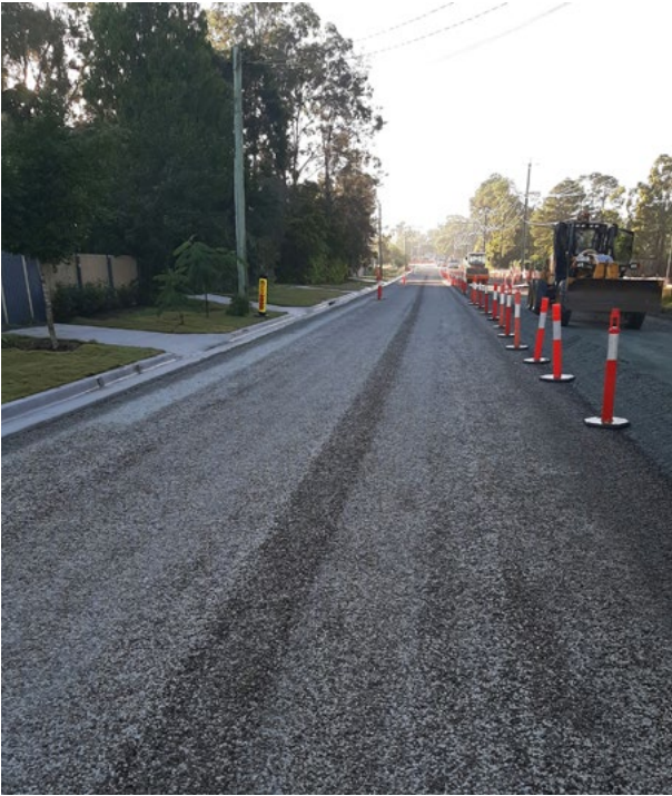
Webb Road – construction
