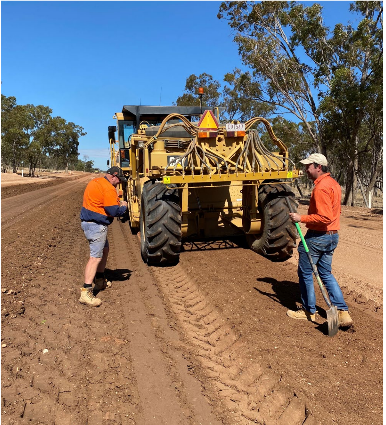
Alpha-Tambo Road – construction
