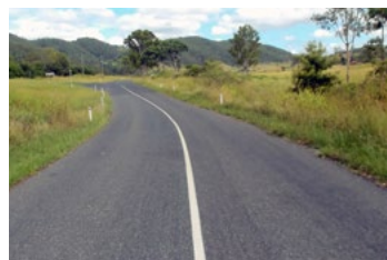
Mary Smokes Creek Road and Sandy Creek Road – before
