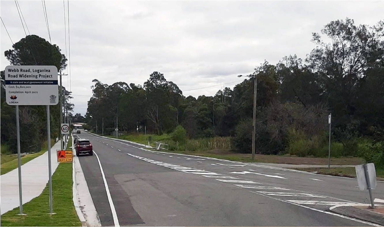
Webb Road – completed
