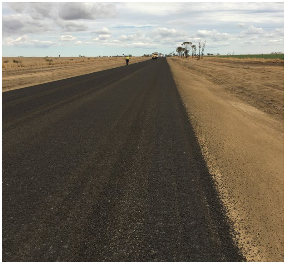
Wyuna Road – after
