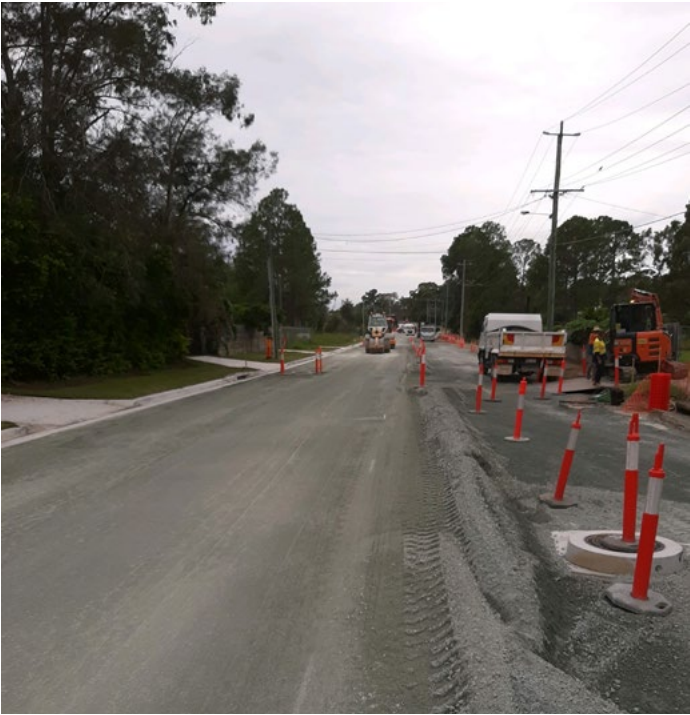
Webb Road – construction
