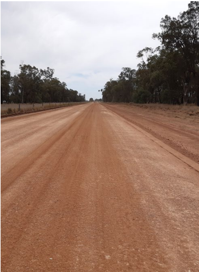
Arubial Road – before
