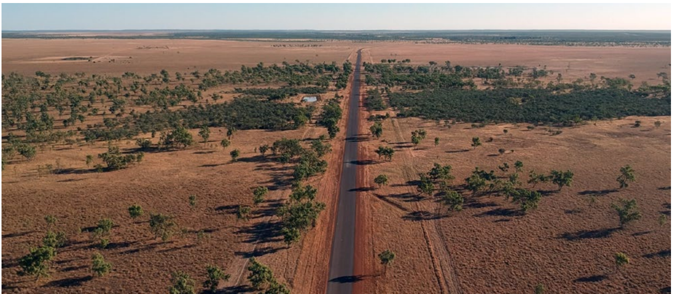
Normanton Burketown Road – completed
