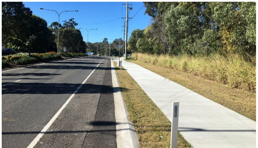
Manly Road – after
