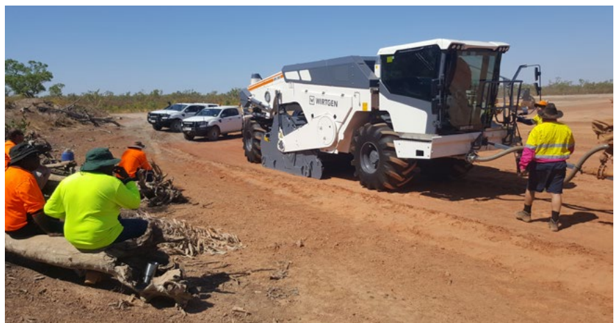
Soil stabilizer and crew
