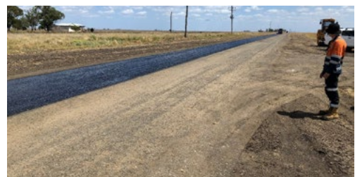
Bongeen Road – construction
