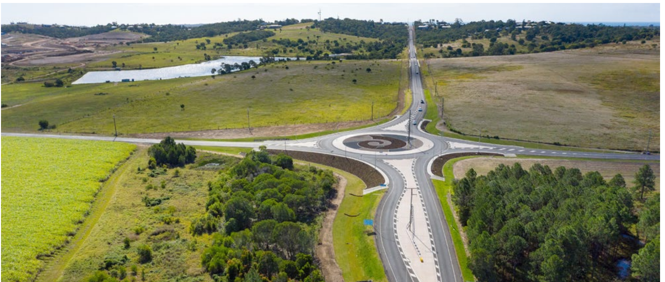
Upgrade of Main Street, Chapel Road and Maggs Hill Road Intersection – after
