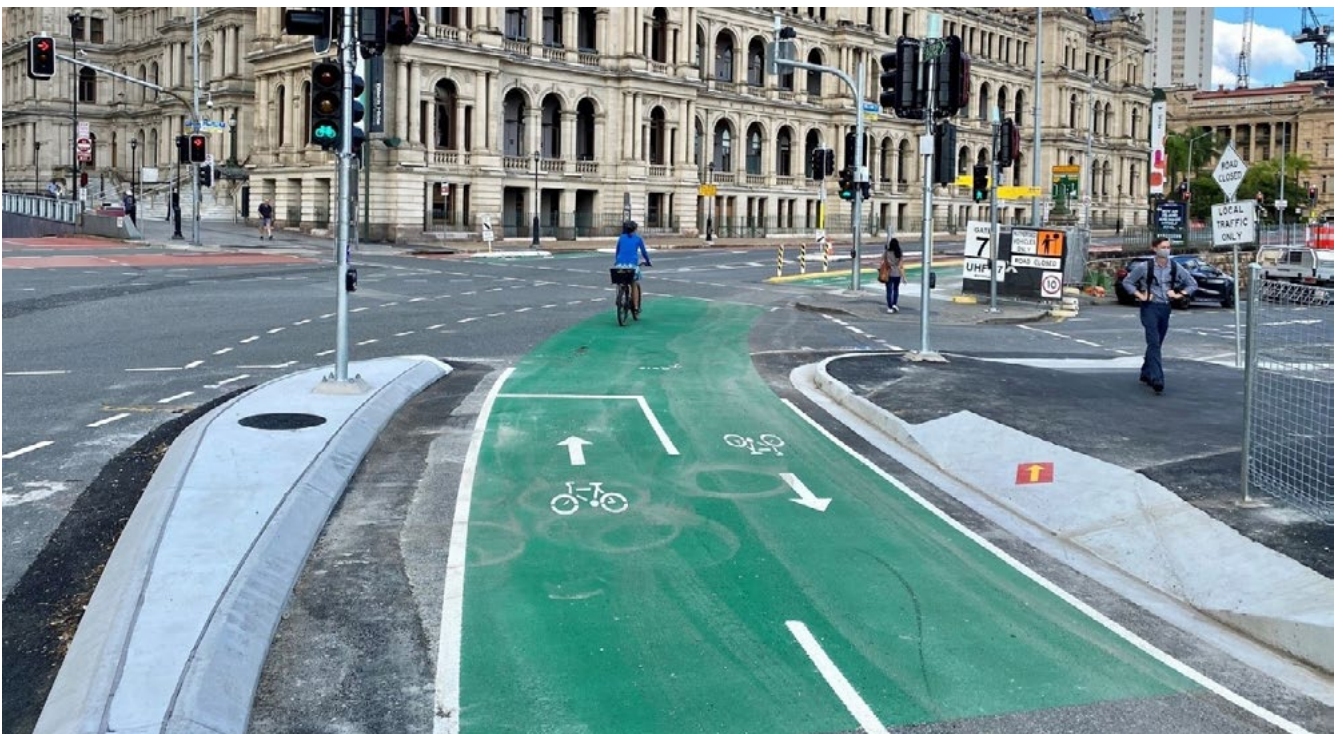
CityLink Cycleway – Stage 2, William Street to Gray Street – after
