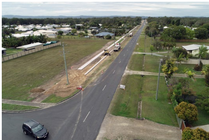
Investigator Avenue – before
