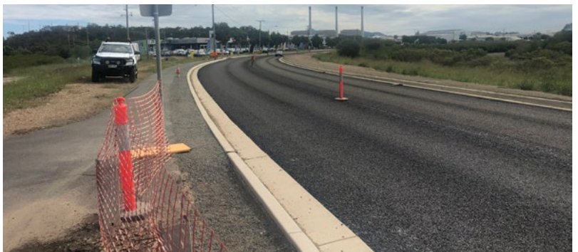
Blain Drive – construction
