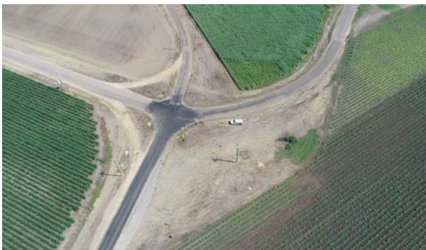
Fiveways Road and Ivory Road Roundabout – before
