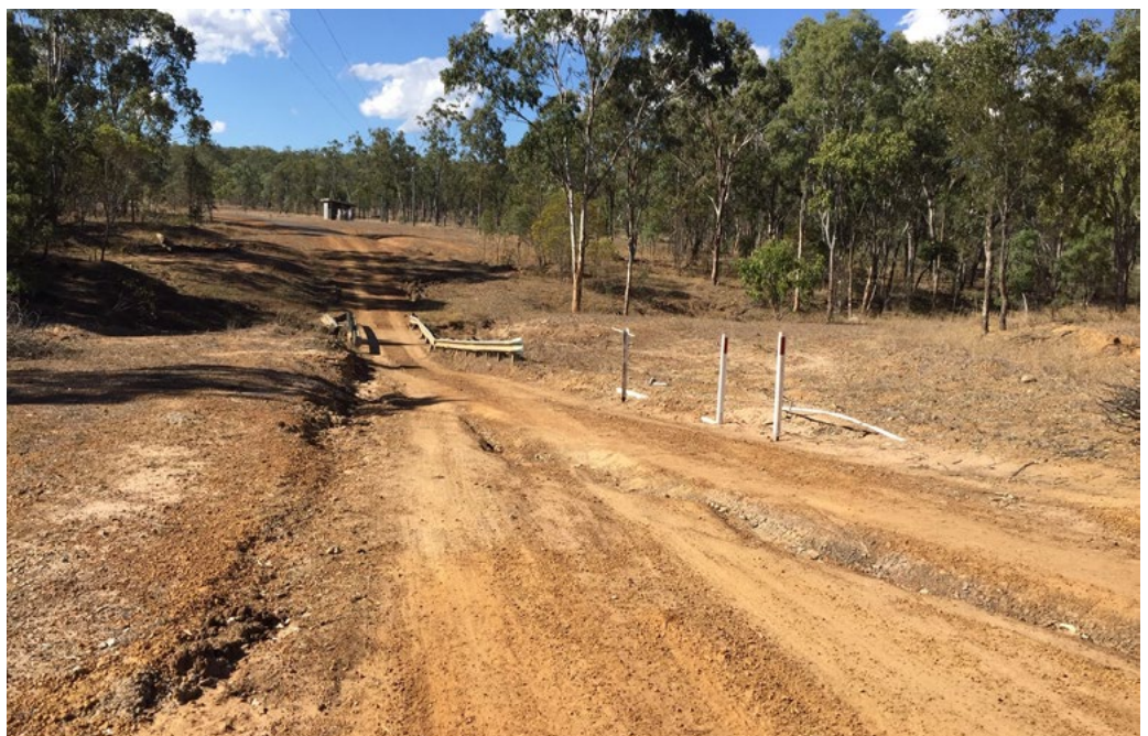
Bore 3 Road, Blackboy Creek Bridge – before
