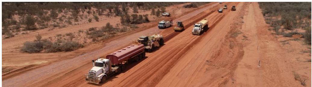
Quilpie-Adavale Red Road - construction
