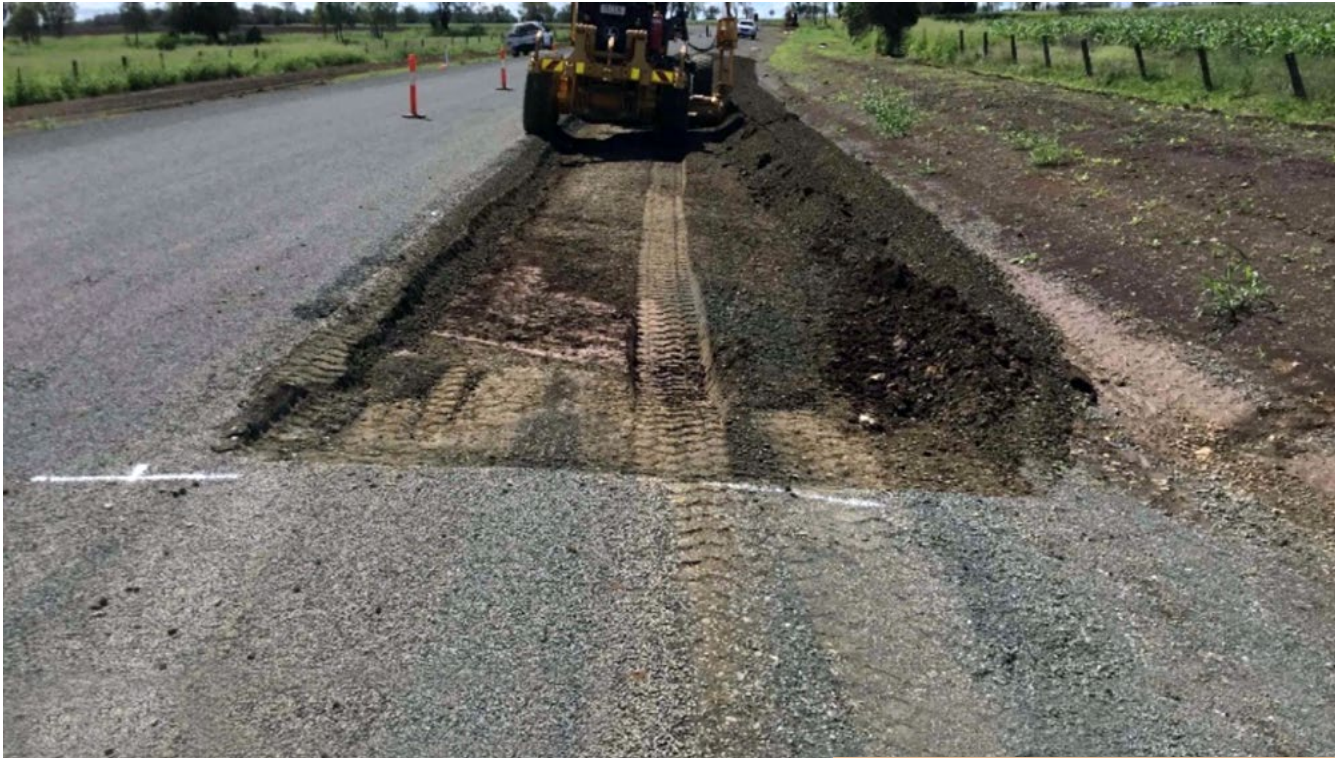
Bowenville Moola Road – repair and reconstruction of wet subgrade
