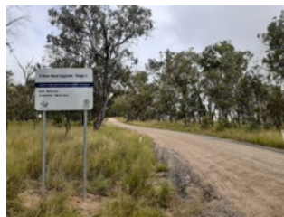
O'Deas Road – before
